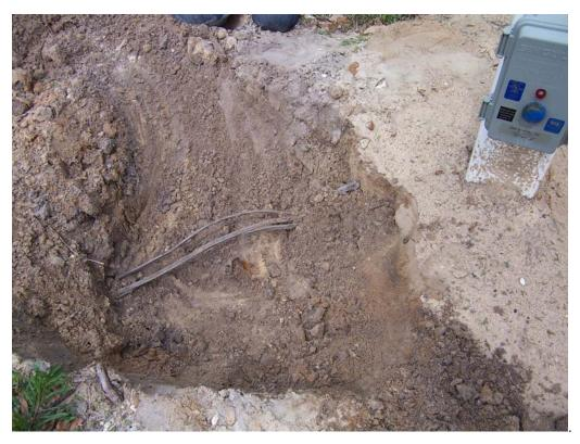
Figure 15. Picture taken on 04/20/09 of Norweco system with wires strung across the pump tank lid preventing access. No sampling port was installed. Maintenance records indicate the effluent was visually inspected.
