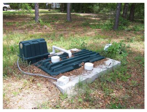
Figure 12. Picture taken on 04/16/09 of a FAST system with the unwired control box lying on the exposed tank. The system was in use with sewage, but no electricity.
