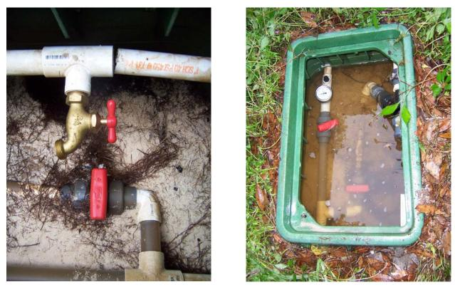
Figure 17. Pictures of site WS-4 taken on April 14, 2009. The broken plumbing evident in this picture was also reported in September 2008. The broken pipe caused the effluent to fill the control box instead of going to the drainfield.
