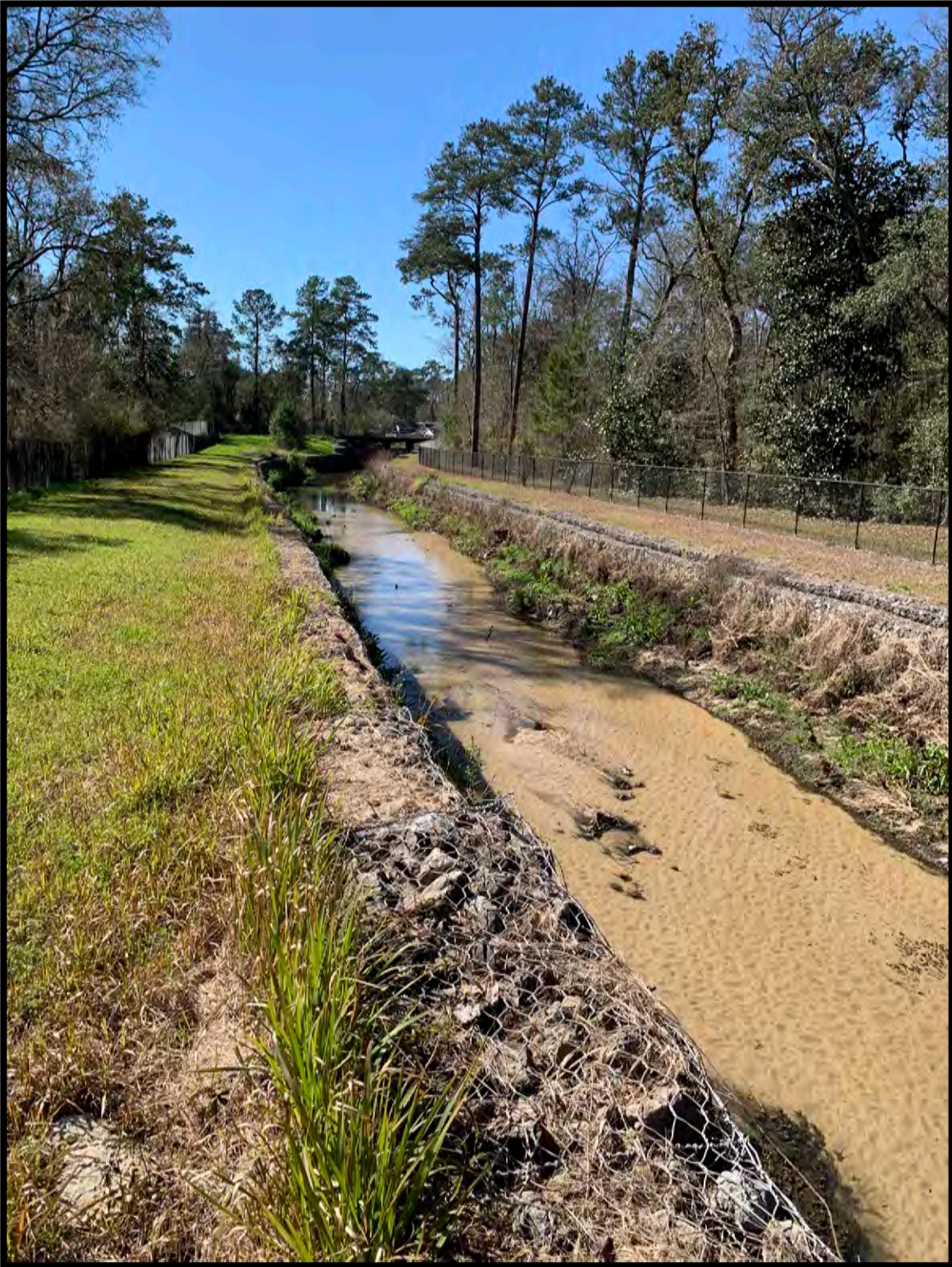
Photo 3-51: Photo of Bank Stabilization along East Ditch West of South Adams Street (2021)
