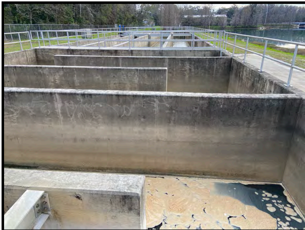
Photo 5-17: Weems Pond Regional Treatment Facility Alum Mixing Chambers
