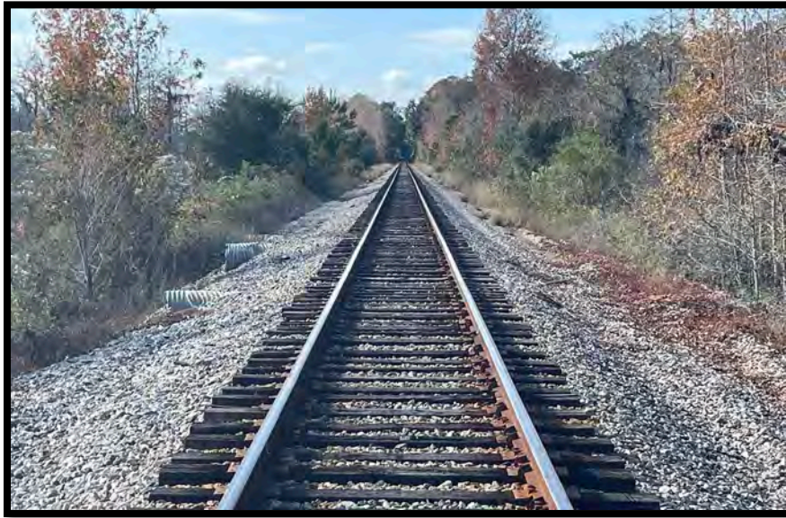
Photo 5-29: High Flow Culverts through CSX Railroad Berm in 2023
