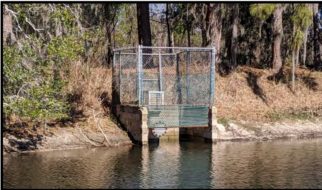
Photo 5-21: Drop Inlet Structure along Western Side of Piney Z Lake Exposed During Low Water in 2020
